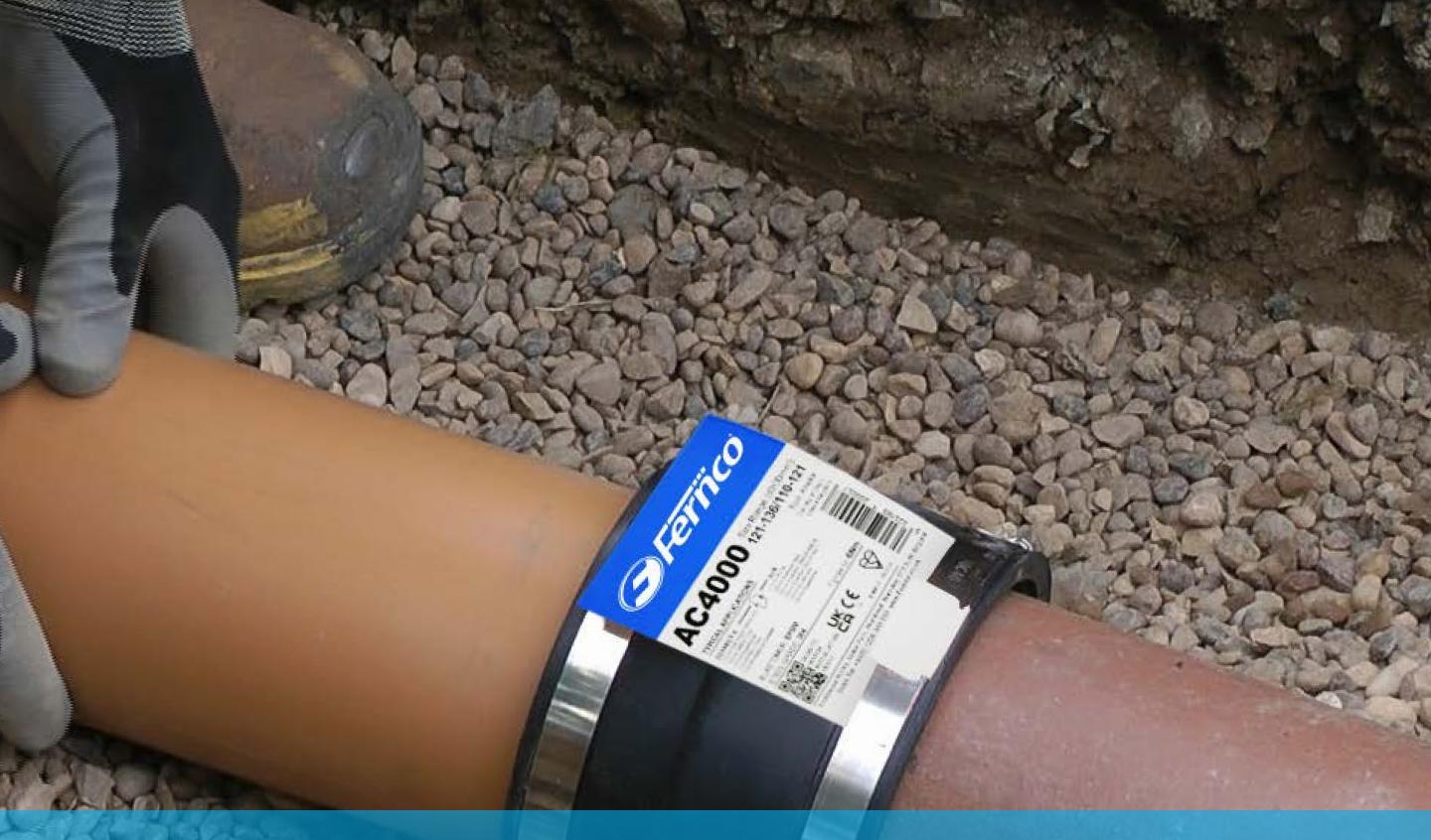
FERNCO ADAPTOR COUPLINGS ARE DESIGNED TO CONNECT UNADOPTED DRAINAGE PIPES WITH DIFFERENT OUTSIDE DIAMETERS.
